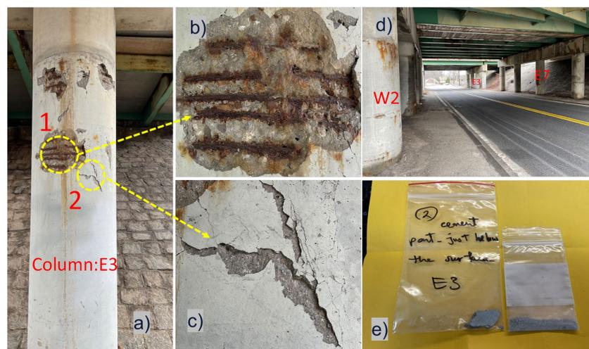
**Fig. 1:** a) One selected bridge pier (E3); b) Enlarged deterioration region (sample collection location 1); c) Enlarged deterioration region (sample collection location 2); d) RC piers of I-495 bridge in Chelmsford, MA; e) Collected samples for characterization
