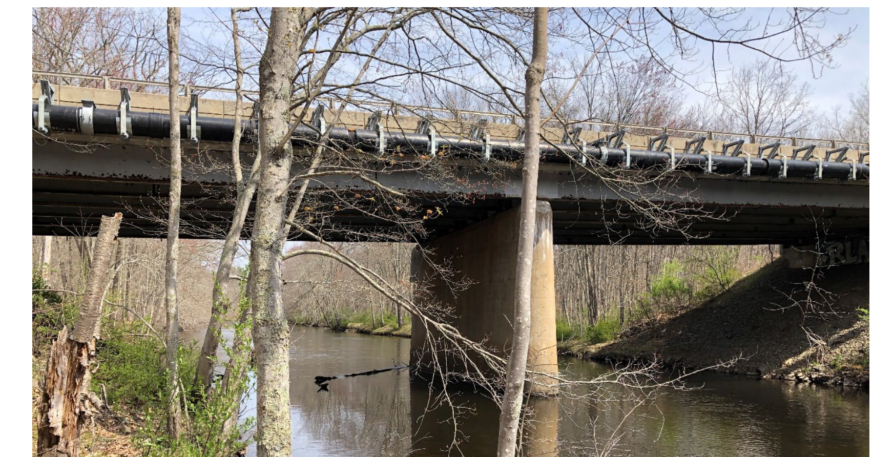
Figure 5. Testbed Bridge in Tolland, CT
