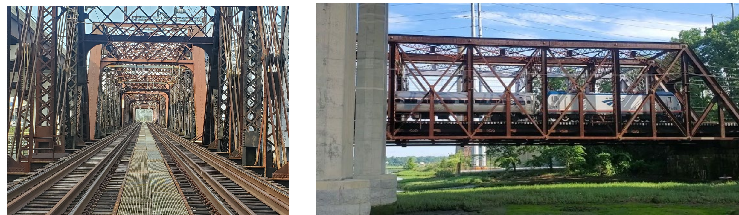
Figure 1: Devon Bridge span 7 th , deck (left), and elevation (right)
