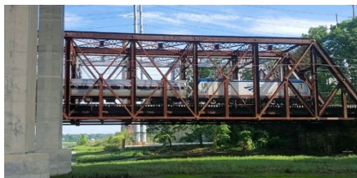
Figure 1: Devon bridge east abutment span
