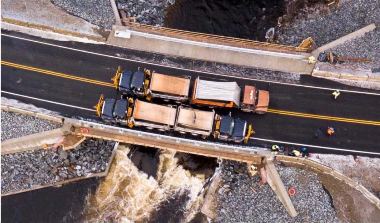
Figure 20: Aerial Photo of MAX_1_1 Test (Courtesy of Advanced Infrastructure Technologies)
