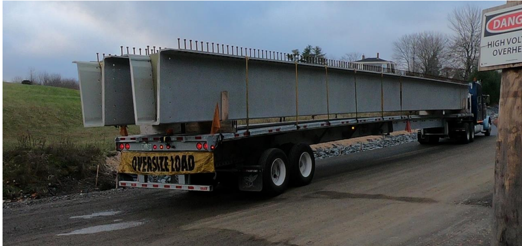
Figure 11: Girders Arriving at Bridge Site
