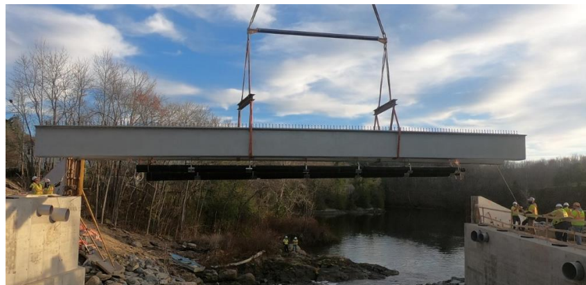
Figure 13: Two-Girder Unit Being Lifted into Place
