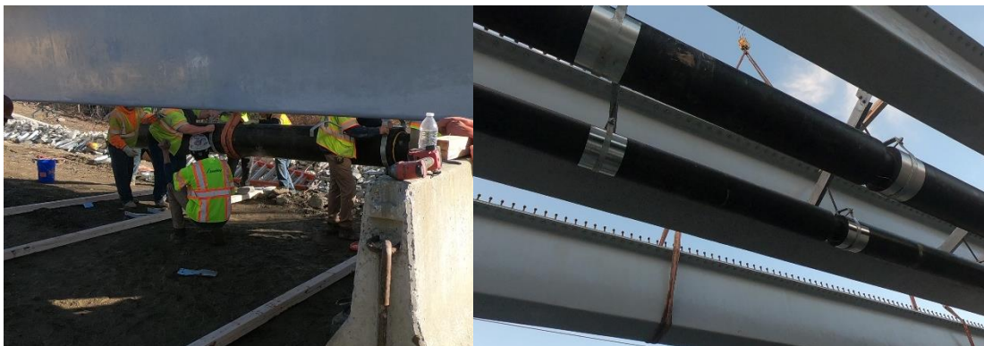
Figure 12: Utility Hangers (Left: Installation; Right: In Place)
