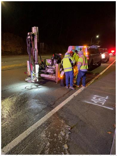
Figure 2. RIDOT's coring crew obtaining cores during the project period at one of the sites where GPR testing was performed for this project.
