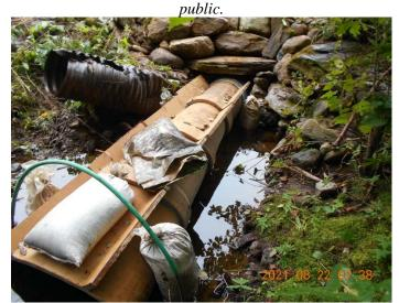
Figure 1. Thorndike, ME, 3D printed diffuser installation
