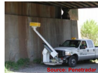
Remote SAR inspection
