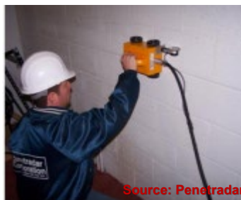
Contact GPR inspection
