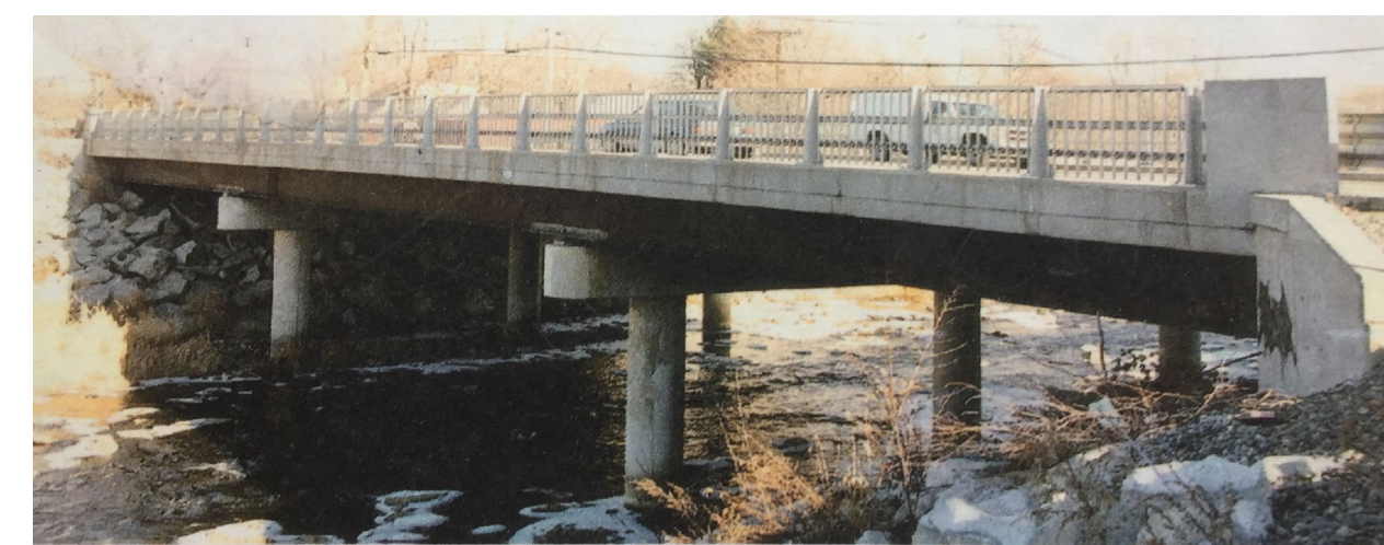
Fig.2 Three span IAB in Fitchburg
