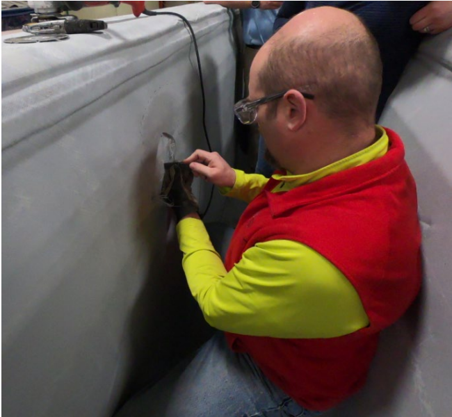
Investigation of Girder Defect
