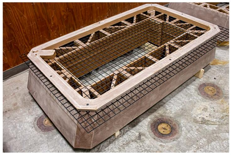
Figure 2. 3D printed form parts for precast concrete panel window opening
