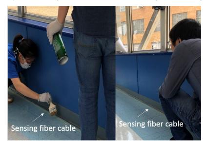
Figure 6: Apply 3M Hi- Strength 90 spray adhesive between the floor and the sensing fiber cable.
