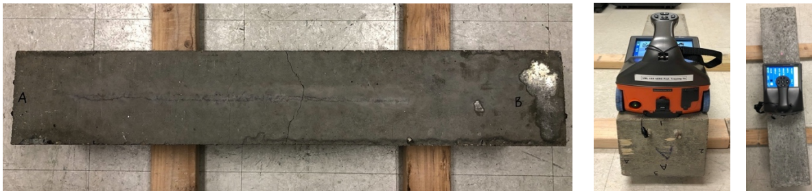
Fig. 1 a) Cracked RC beam specimen
