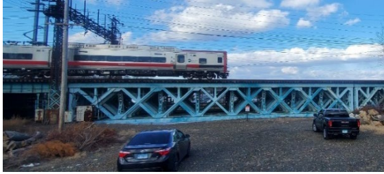
Figure 1 – Cos Cob Bridge: Train 4 during tests
