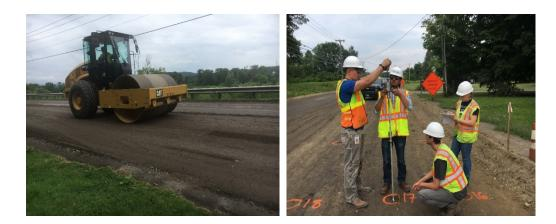
(a) (b) Figure 1: IC compaction in the field, (b) Performing DCP test
